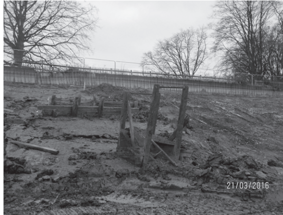
In the Model Boating Pond underneath the area of the new dam: 19 th century oak revetments and, in the foreground, the remains of the entrance frame for the (still extant) underground pipe into the downstream Men's Bathing Pond.
