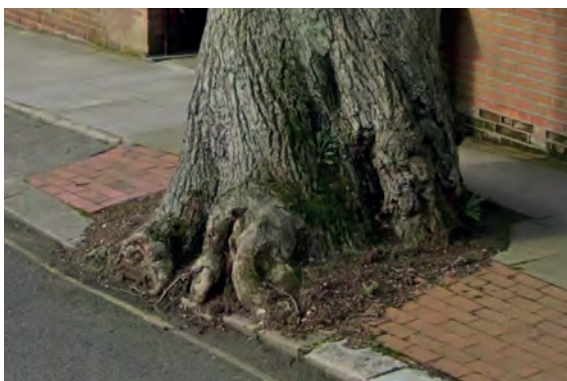
Base of tree with granites 'flowed over' and vehicle impacts (2018)
