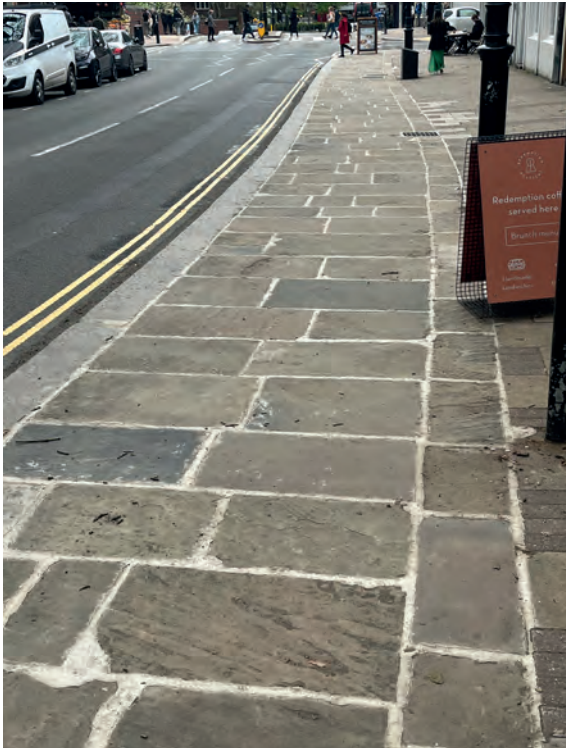
The reclaimed York stone in the new streatory in South End Road
