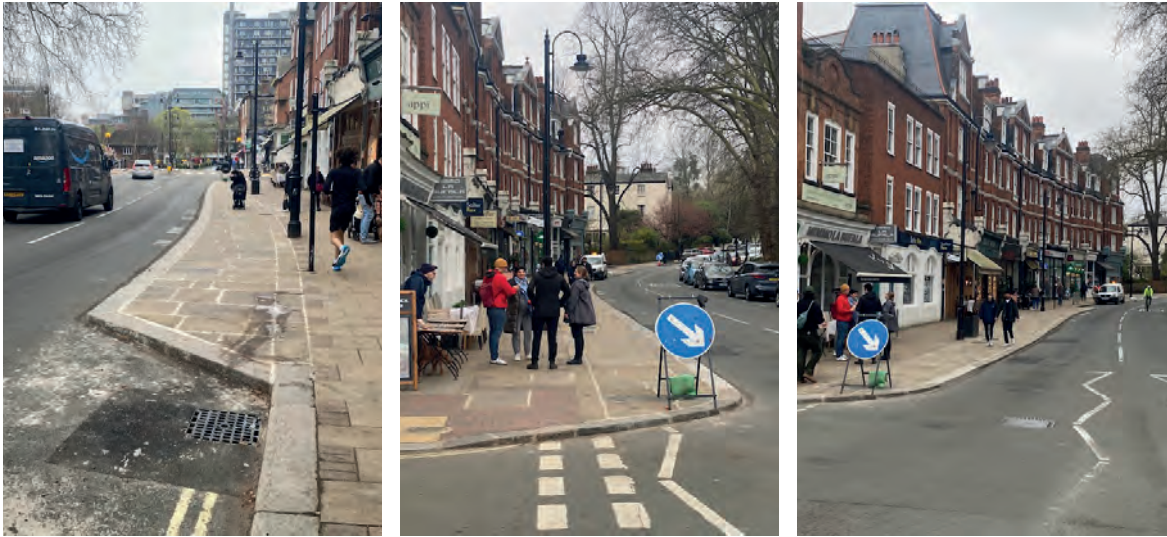
Views of the build-out of the pavement with York stone on South End Road, already contributing to the comfort of pedestrians
