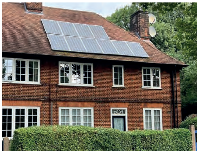
Example of solar panels on a clay tiled roof
