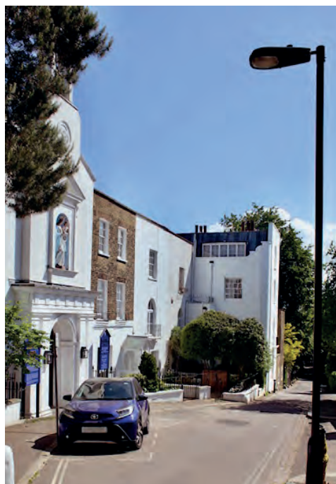
Victorian lamp replaced in 2025. St Mary’s, Holly Walk
