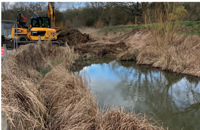
Digger at work
